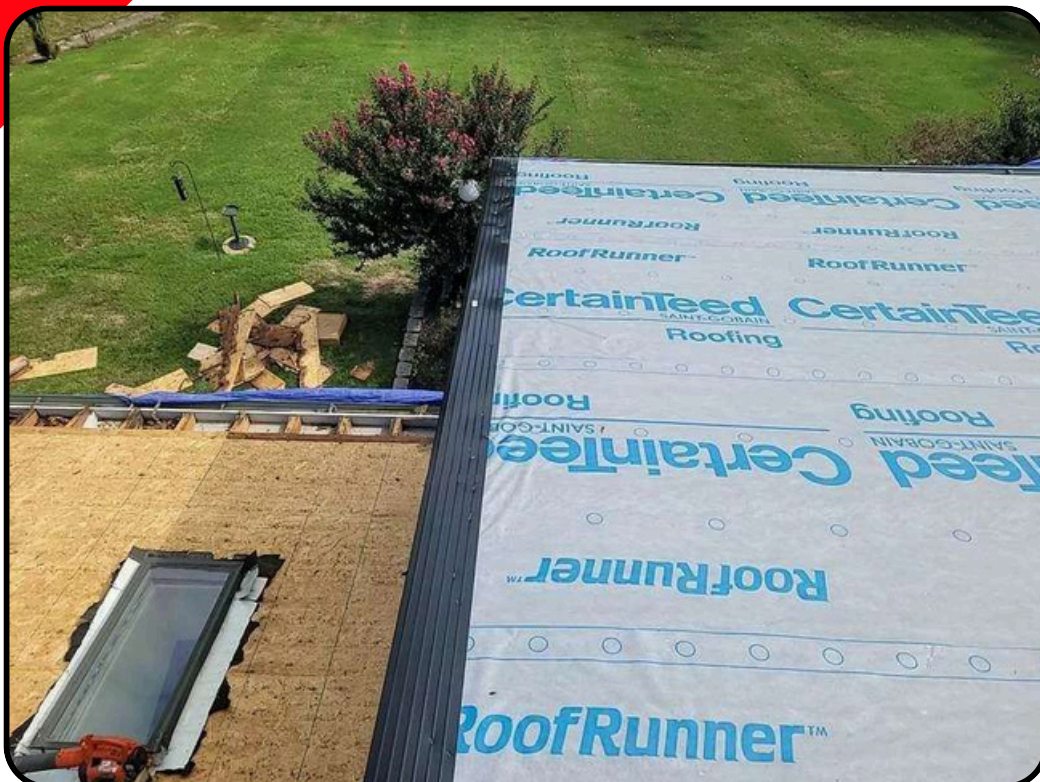
↑ EXAMPLE OF STANDARD DRIP EDGE
