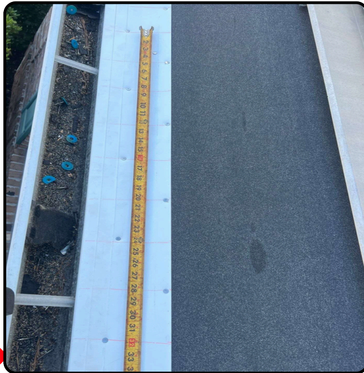
↑ FORTIFIED DRIP EDGE NAILING PATTERN
