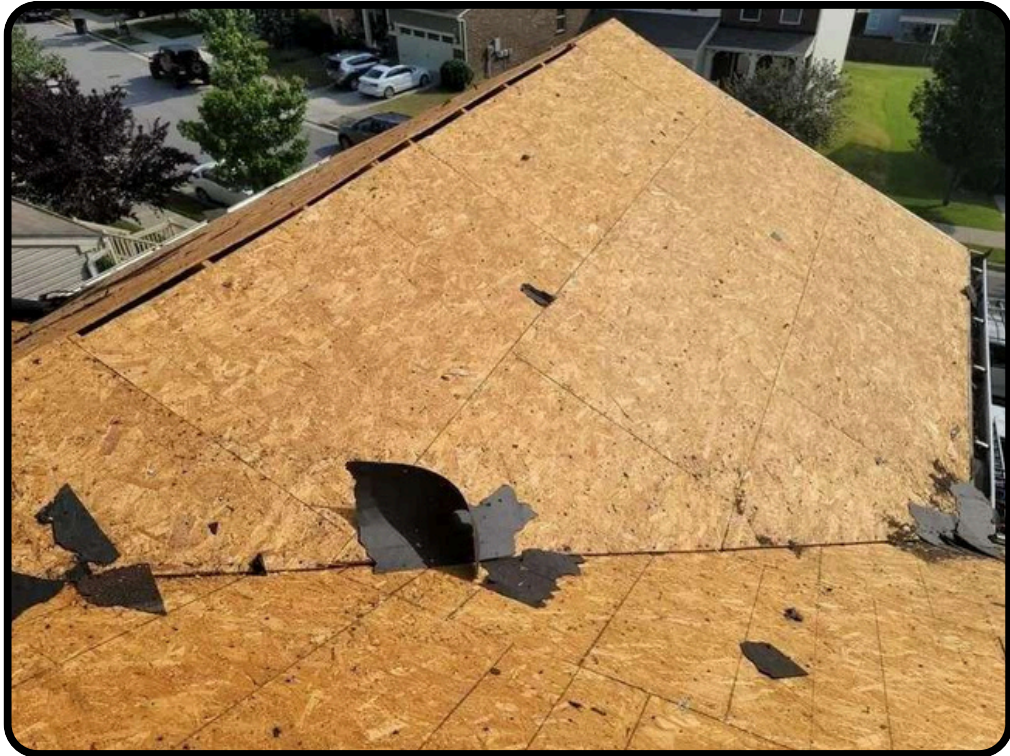
↑ EXAMPLE OF A ROOF DECK THAT WAS STRIPED DOWN
