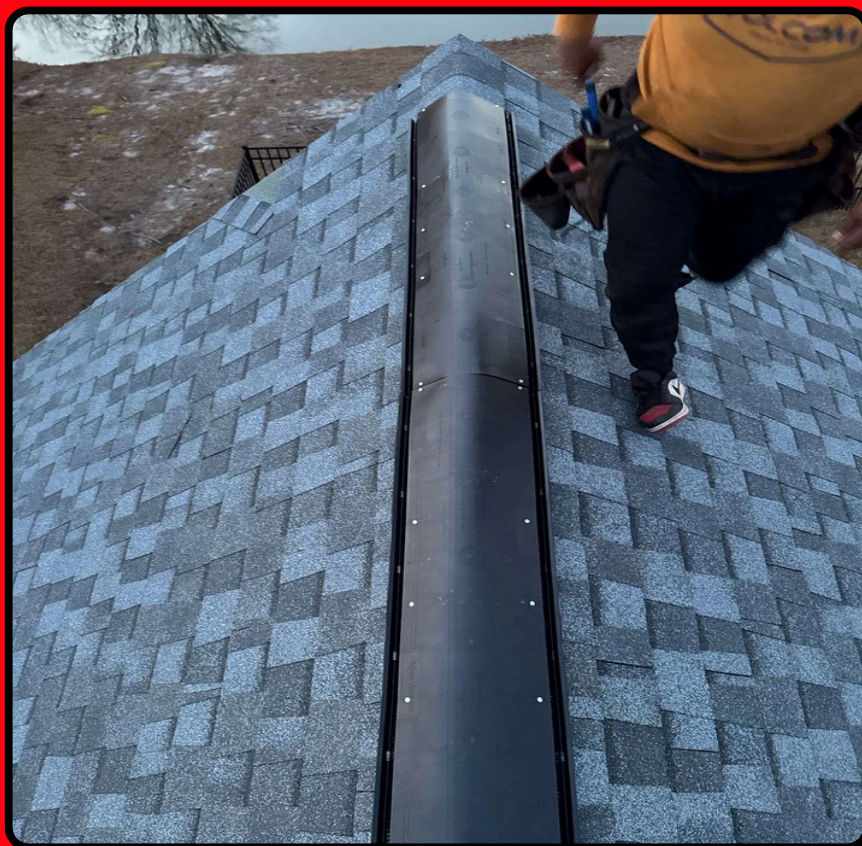
↑ Example off an upgraded ridge
